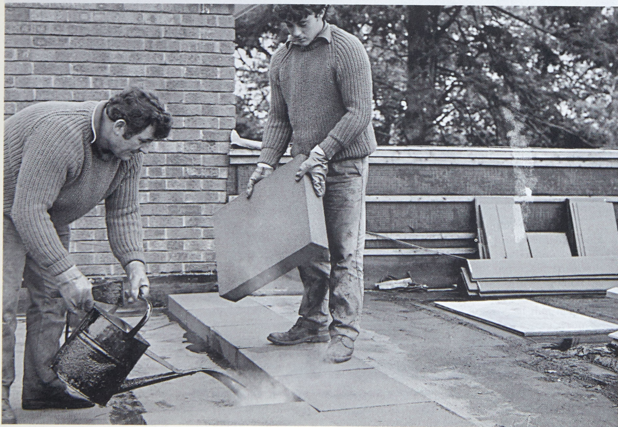
Workmen placing blocks of Foamglas on the new roof.
